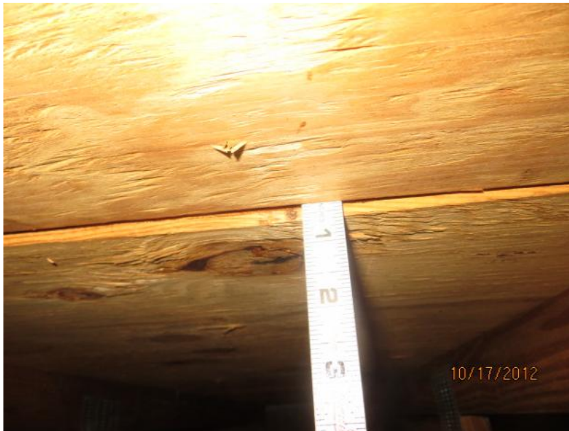
5/8" Deck Thickness Confirmed
