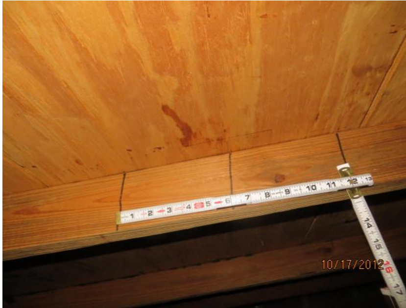
8d Nails Spaced 6" Along the Edge
