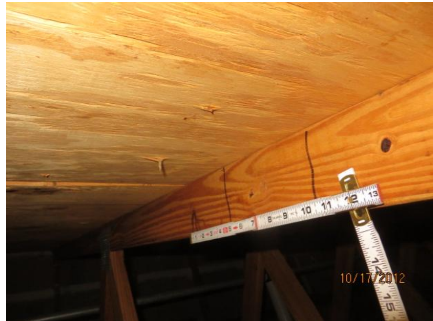
8d Nails Spaced 6" in the Field
