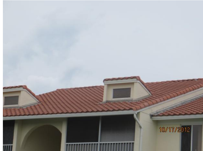
Concrete/Clay Tile Roof Covering
