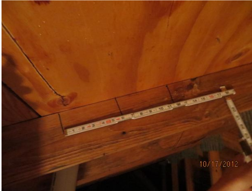
8d Nails Spaced 6" Along the Edge
