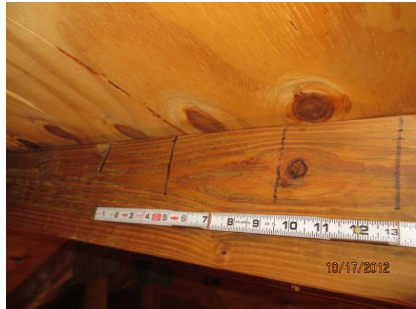
8d Nails Spaced 6" in the Field
