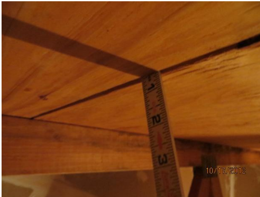
5/8" Deck Thickness Confirmed
